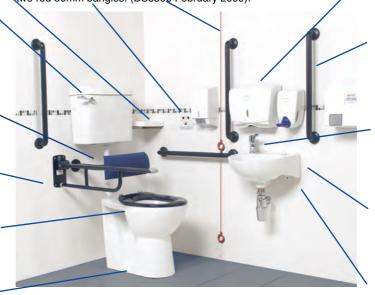
Two clothes hooks, one should be positioned at 1050mm and the other positioned at 1400mm above the floor. Stainless steel mirror 1000mm x 400mm. The above items are fitted on the opposite wall to the basin.
